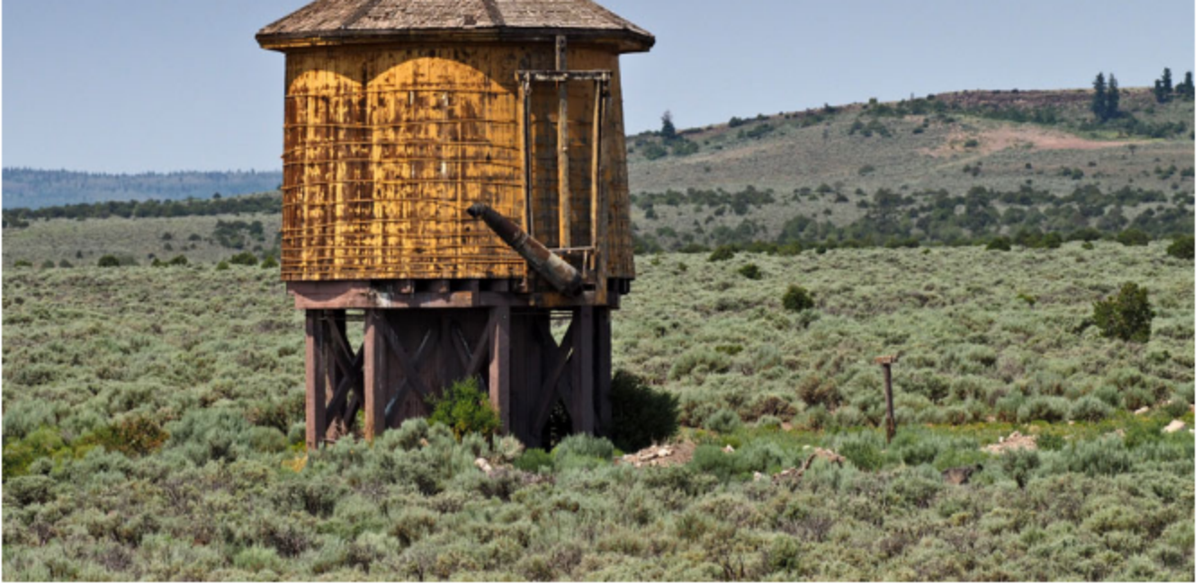
This water tower at Lava was originally located in Antonito, but was moved here after the original tower burned in 1971. It is not currently in service.
