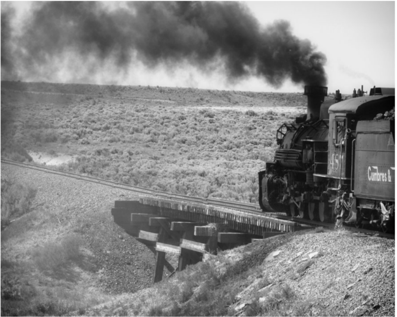
This low trestle is known as “Hangman’s Trestle” because some vigilantes “borrowed” a locomotive from the Antonito yard and hung a Mr. Ferguson at this bridge for an unknown crime.
