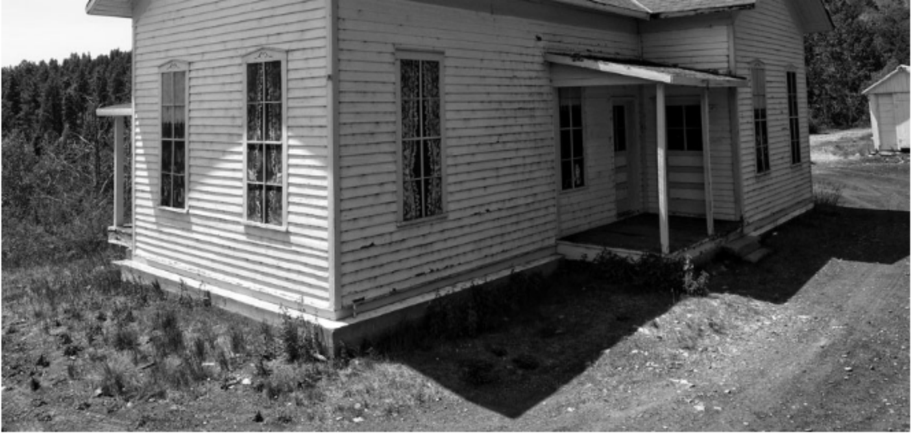
This is one of the section gang houses at Sublette. Note the “curtains” in the windows, they are actually just painted onto boards over the windows!
